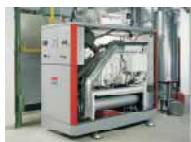
▶ BHKW Sokratherm 50 kWel
