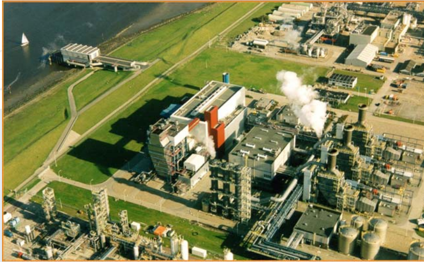
Akzo Nobel: Delesto CHP plant. It provides steam and power to Facilities in Delfzijl where Akzo Nobel produces salt, chlorine and Derivatives. It produces 520 MW of power.
