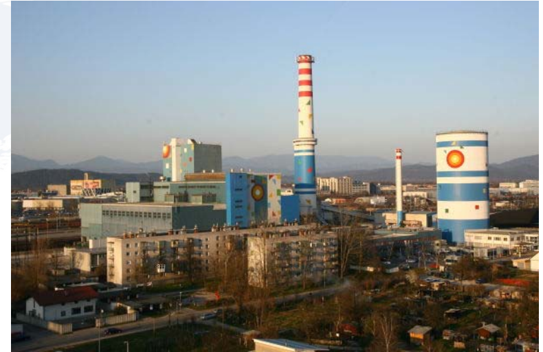
District heating CHP plant in Ljubljana
